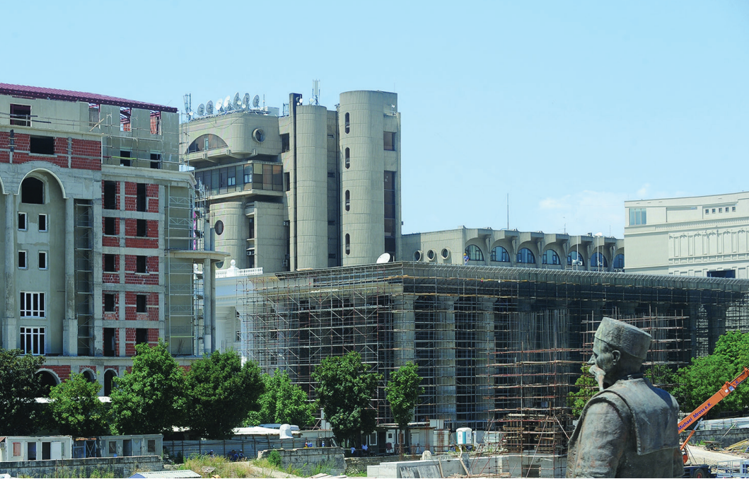
Fig. 7: View towards the Telecommunication Center, 2016
