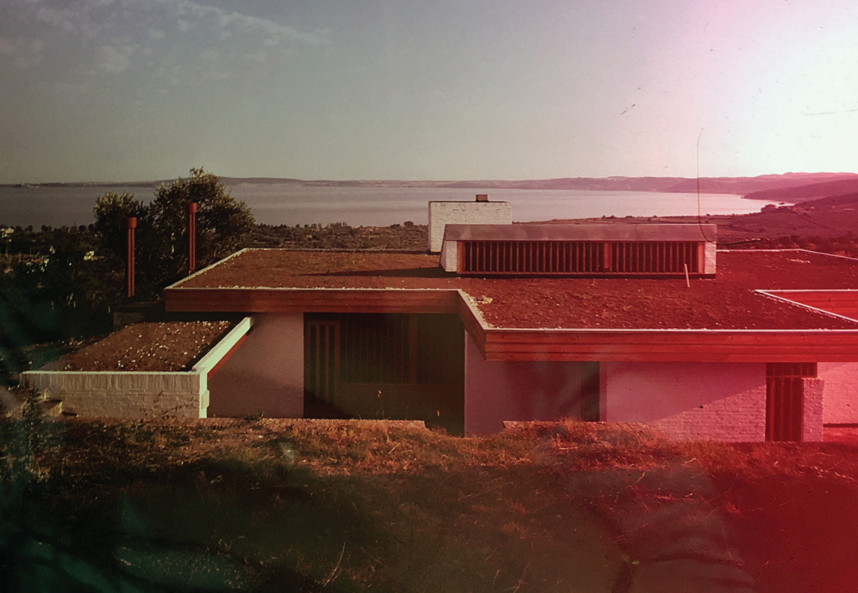
Fig. 3: Villa Rubino/Pedersen and the Lake View seen from the forest at the end of construction (1960s)
