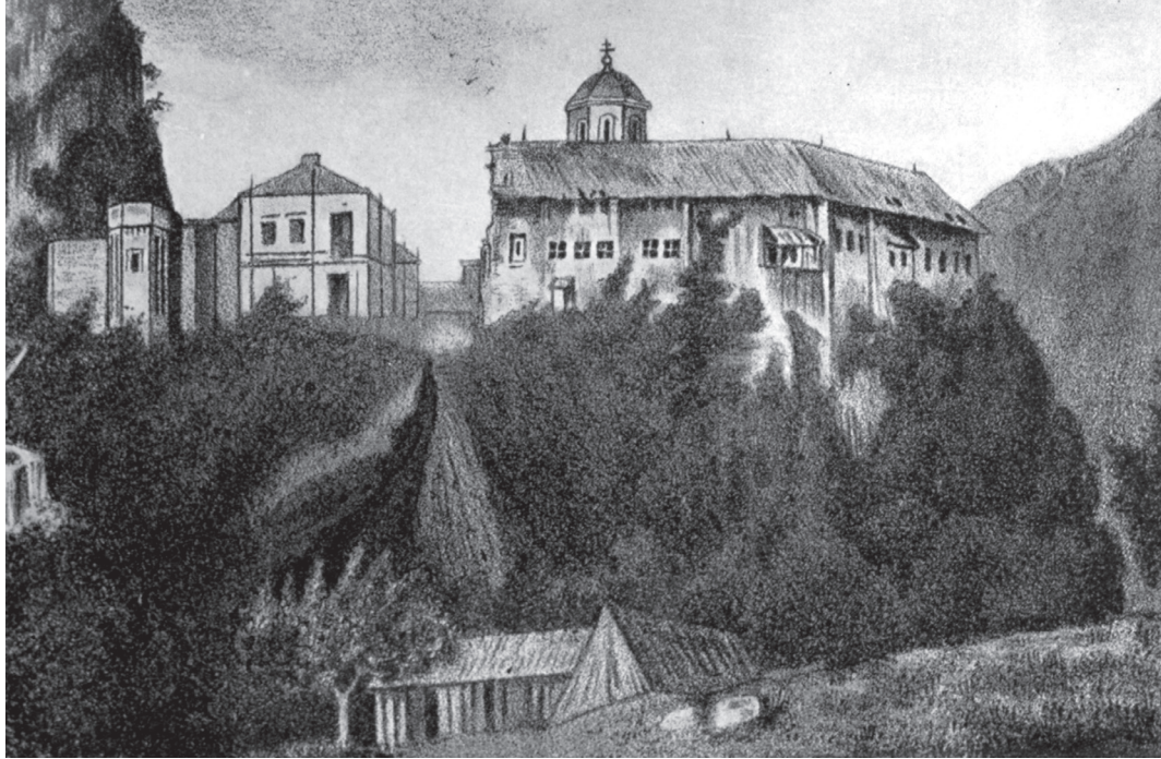
Fig. 1: Tismana Monastery as seen from South-East before the beginning of the restoration works in 1847.
