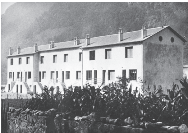
Fig. 23-25: Building in Rioupéroux, photographs showing the construction progress - Livet-et-Gavet, Isère, France
