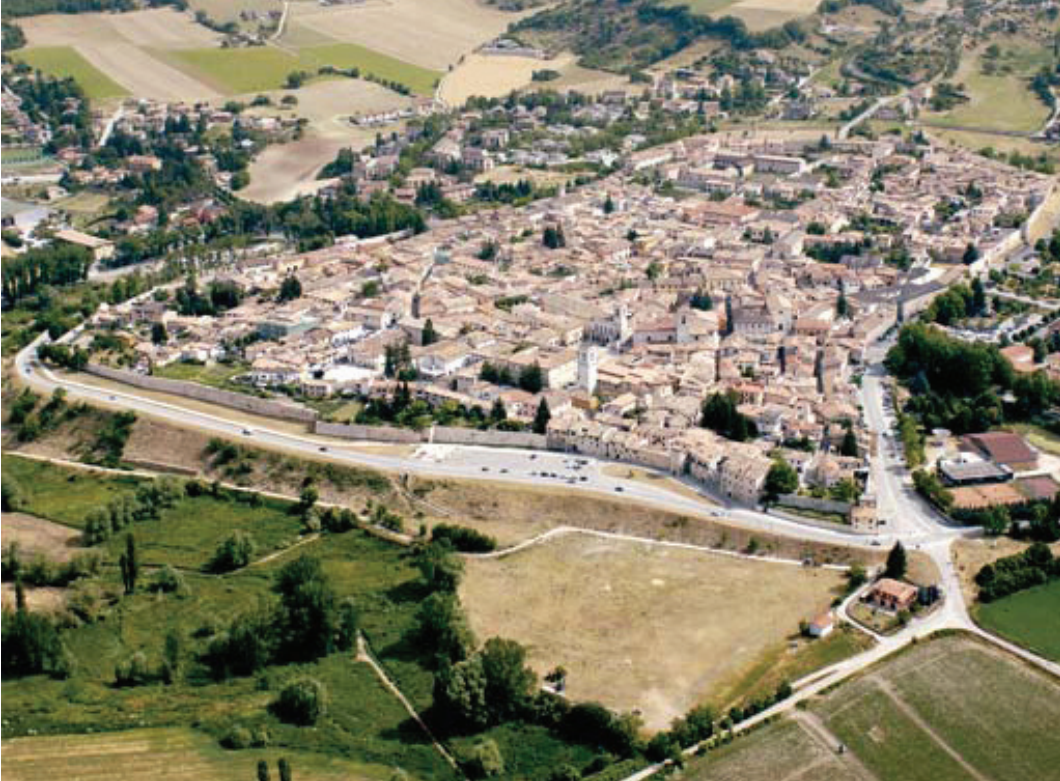
Fig. 03: Norcia, view of the town before the recent earthquake.
