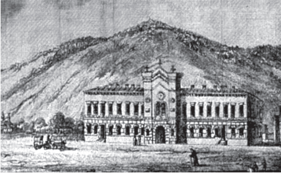
Fig. 3. Alexandru Costinescu – View of “St. Demetrius” hospital in Târgu Neamț in 1882 (still existing), designed in collaboration with architect Ioan (Johann?) Fux in 1852 “...in a beautiful modern Byzantine style” ( Gazeta de Moldova , XXV (1853), 2), actually a Rundbogenstil interpretation of various medieval and classical elements
